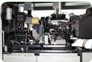
Vacuum and high pressure system are driven by an industrial diesel engine
