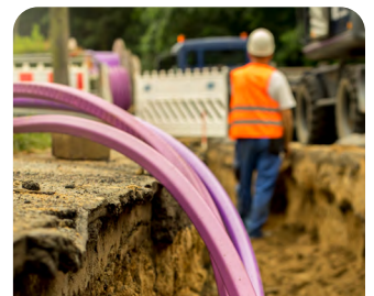
12 to 14 bar: Cable blowing and drilling
