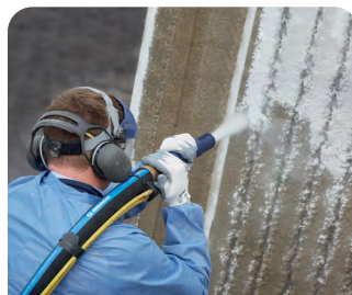
8.6 to 10 bar: Abrasive blasting
