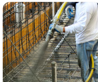
7 to 12 bar: Shotcrete applications
